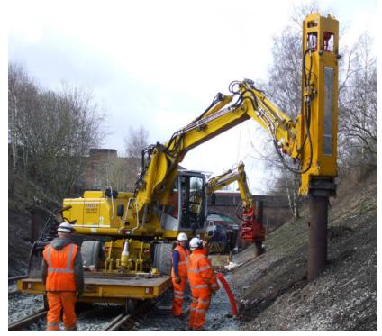
The DX-RT piling hammer is adapted for use on Railway infrastructure applications. Operating from small Road-Rail Excavators of approx 30T mass and above.:
