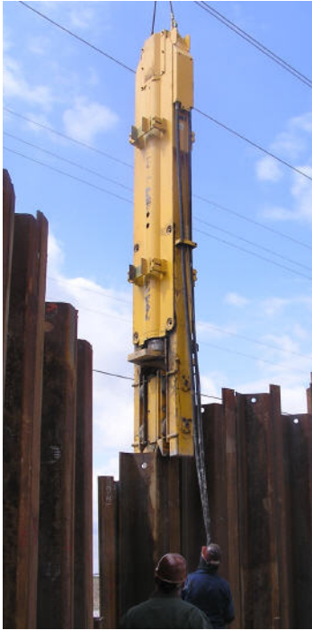
SL30 Hammers fitted with legs and inserts for diving sheet piles.
