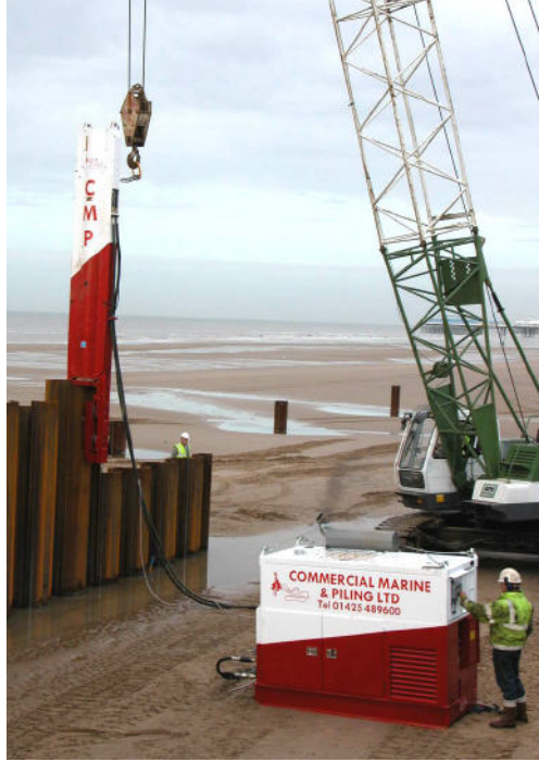
SL30 Hammers fitted with legs and inserts for diving sheet piles.
