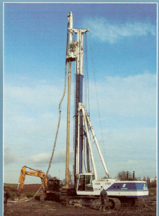
E25 HD-CFA 240 with soil displacement tool
